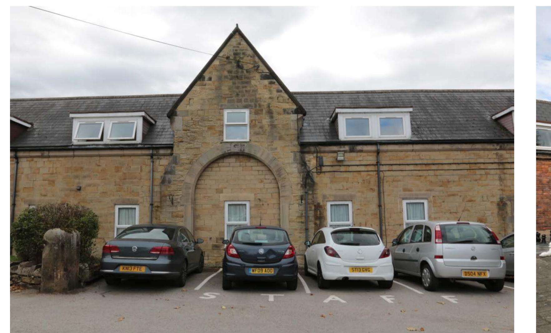
Filled in archway in the original stone faced, north facade
